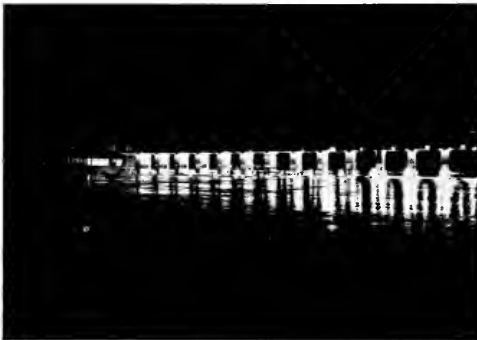
The wet pavement of the Tunnel toll plaza shines after a night rain. There are fourteen toll booths. The Administration Building, headquarters of the Toll Facilities Division, is in the left background.
